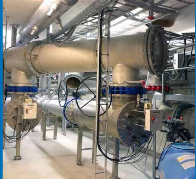
Two Spektron 650e UV disinfection systems.
